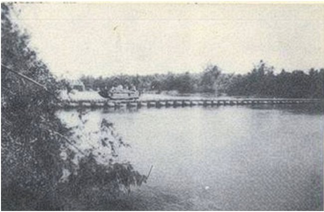
Pontoon bridge completed by the 530th Engineer Light Pontoon Company. Philippines, 1945.
